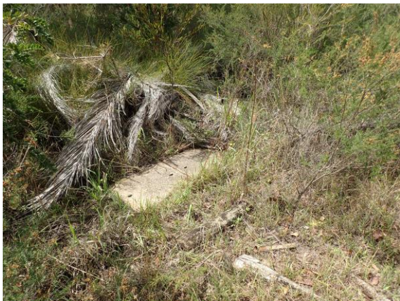
Figure 6.13 Cement man hole cover between the drainage lines. View to south east.
